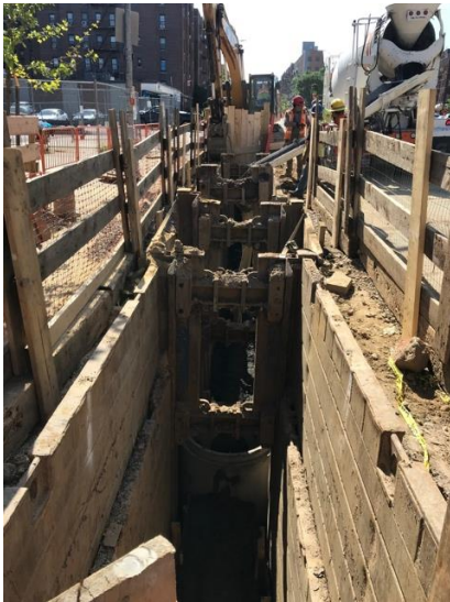
Sewer Upgrades along Empire Boulevard, between Utica Avenue and Schenectady Avenue
