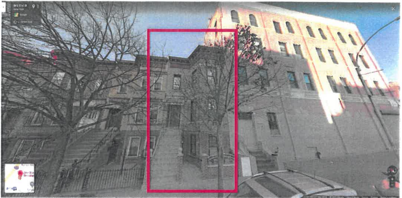
369 51st Street, Brooklyn Existing Building
